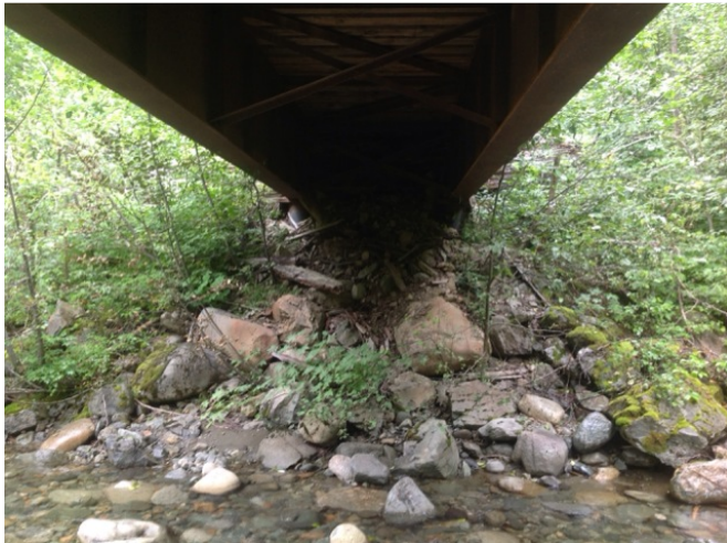
Right Bank Abutment when facing downstream
