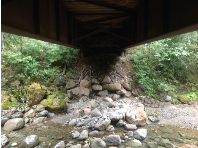
Left Bank Abutment when facing downstream
